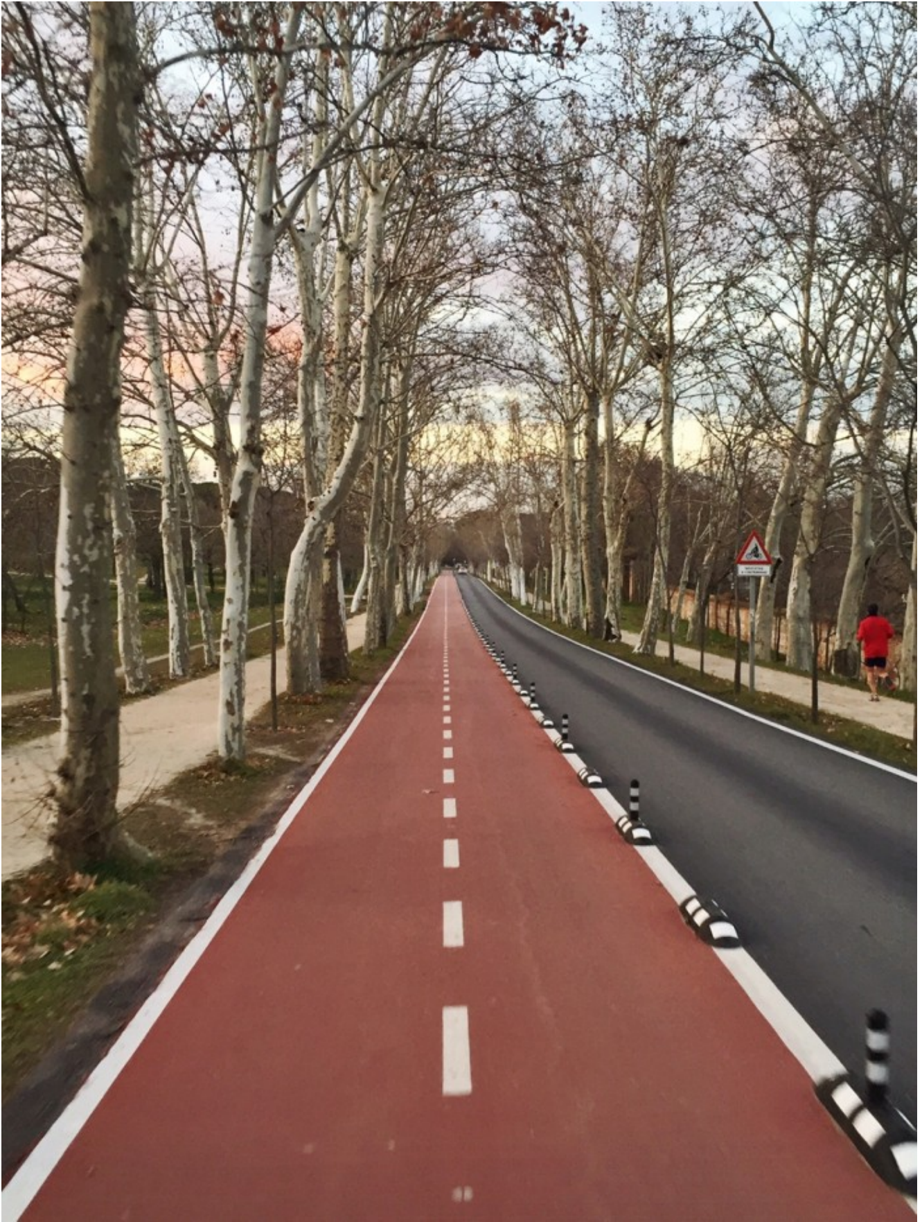
This new bike lane, cutting through Casa de Campo, is part of a growing push by the ayuntamiento to normalize cycling in the city and expand the existing infrastructure.
